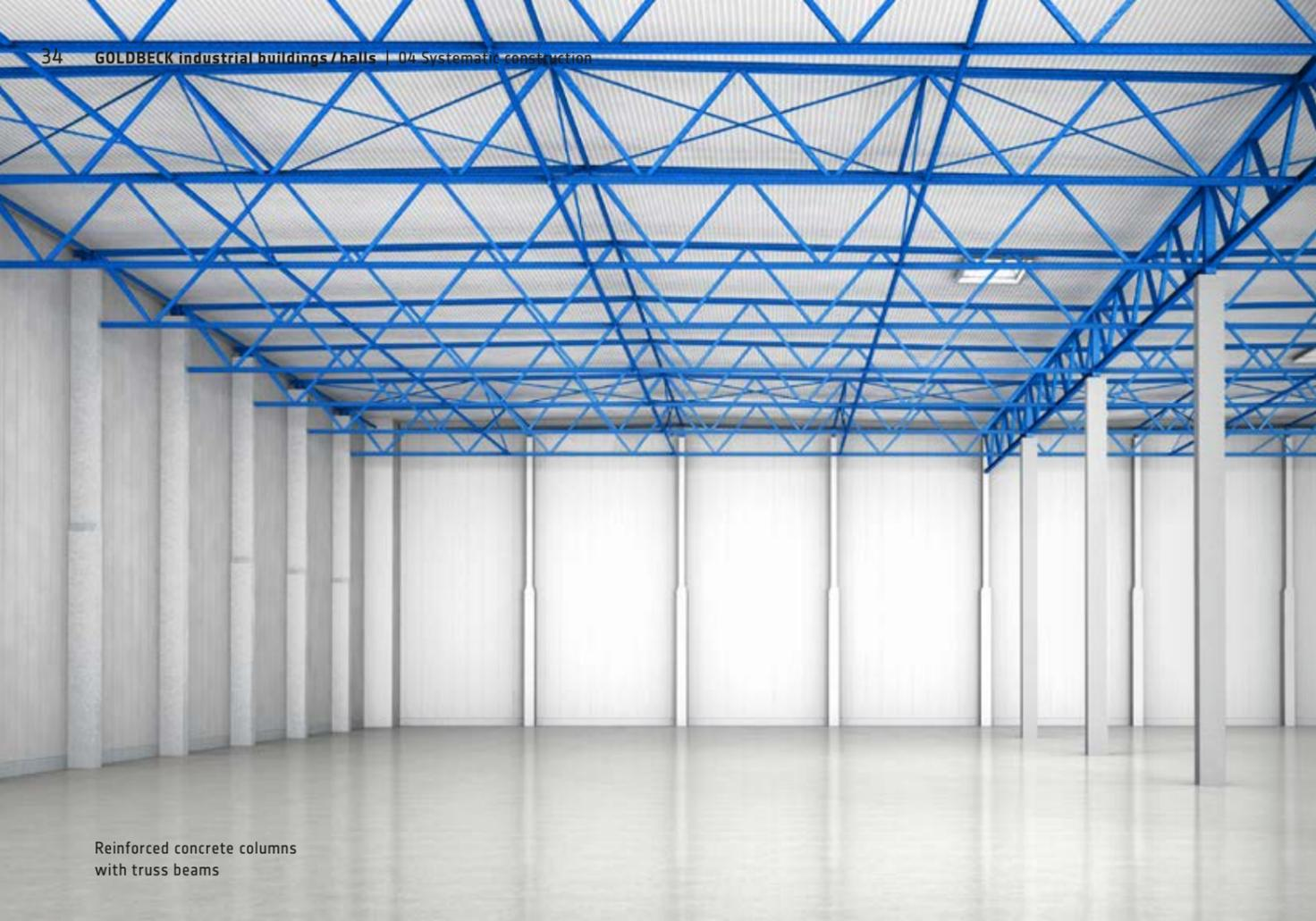
Reinforced concrete columns with truss beams
