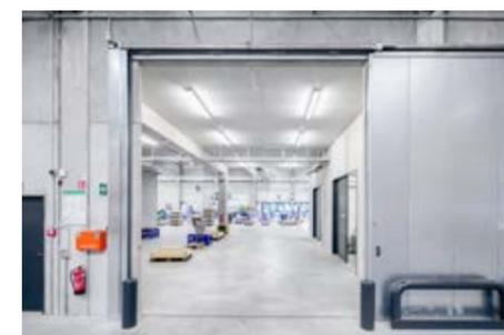
Refrigeration cell, clean room, mezzanine and sliding fire protection gate
