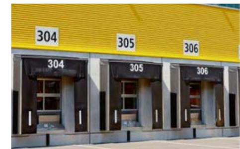
Continuous vertical/horizontal rooflight, sectional gate und loading technology
